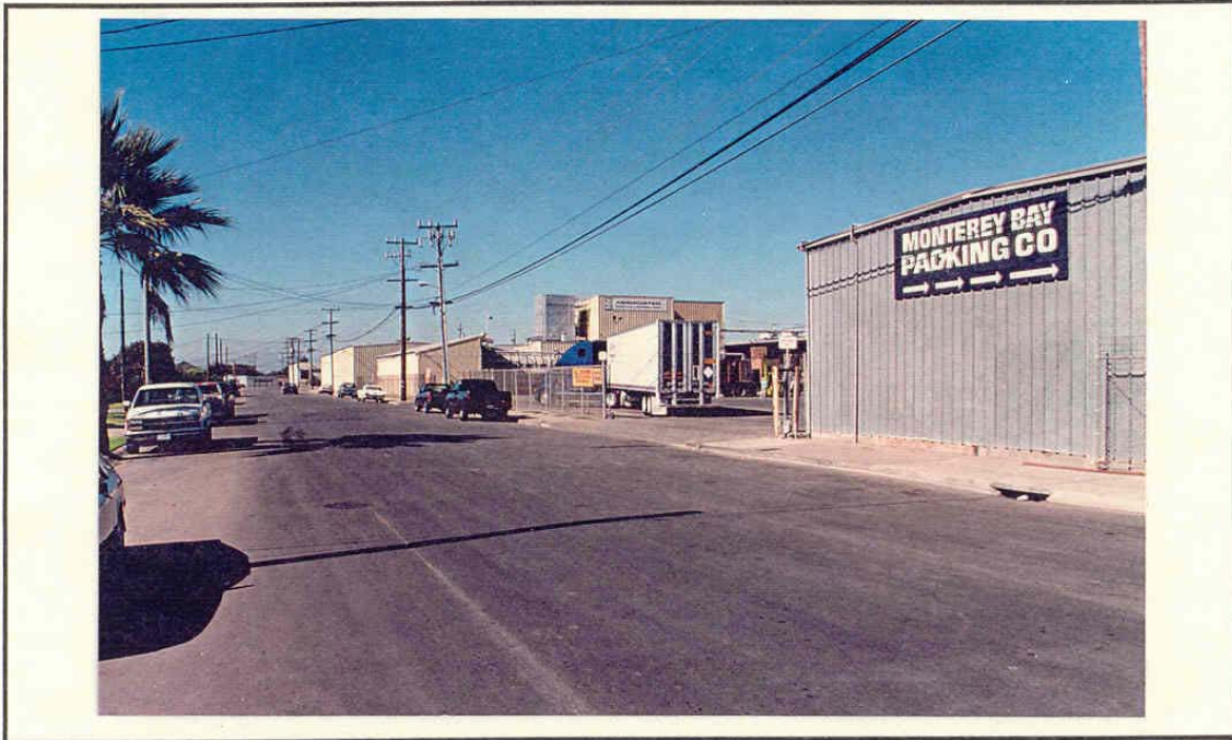
Castro Street frontage and entrance. Shop building and Ice plant in center of photo. California Artichoke plant in background.
