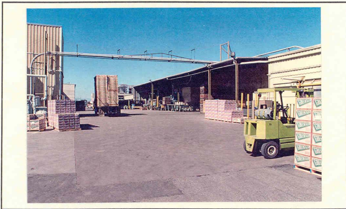
Western elevation of Bldg. "A" and receiving area.
