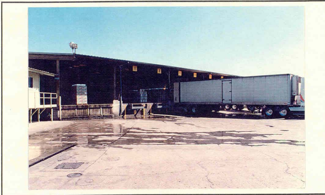
Covered shipping dock.
